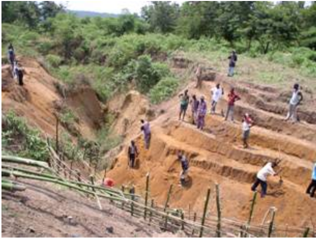
Slope preparation on the left, and the final product after 4 months on the right with the Alain Ndona (right of the sign) who worked with the community on this gully reclamation.
