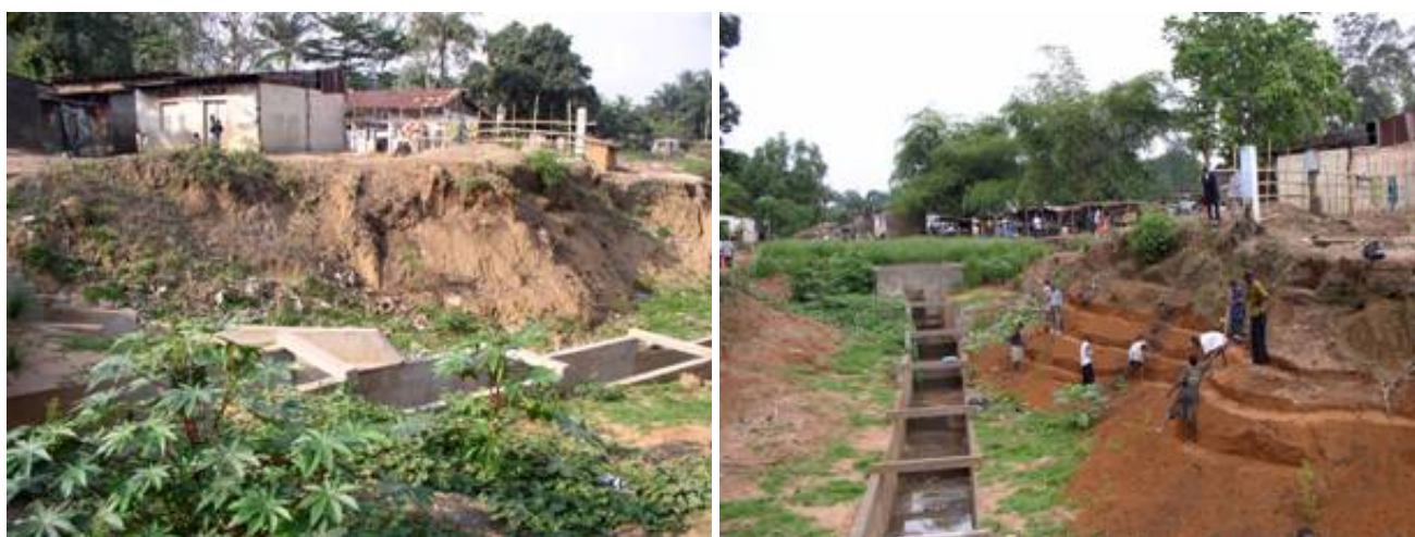
The upper end of the gully threatening the town. The picture on the right shows the gully head already stabilized with vetiver and the slopes being prepared for planting.
