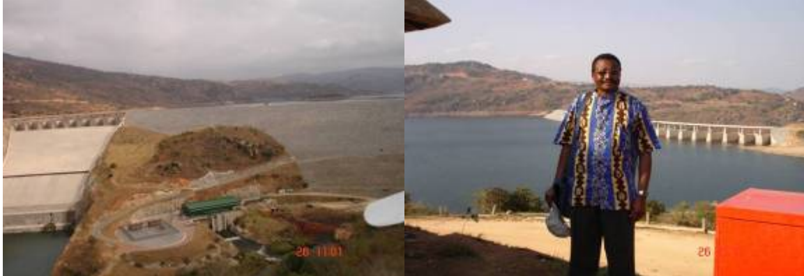
Left: Downstream side of the Maguga Dam showing the spillway and power generation plant (Green building). Right: I am standing on the Upstream side of the Maguga Dam with the reservoir in the background.
