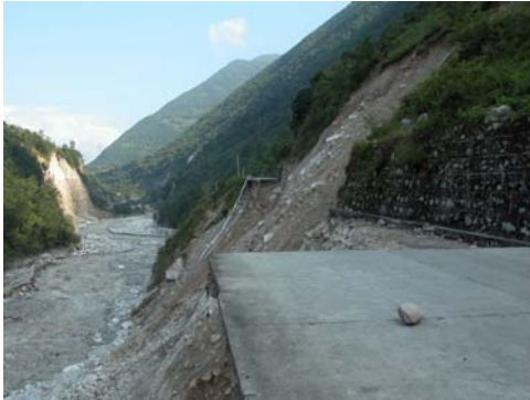
Debris flow rushing onto the road in the Hailuo Gully National Park , by Cui Peng , Institute of Mountain Disaster and Environment, Chengdu, China. pengcui@imde.ac.cn
